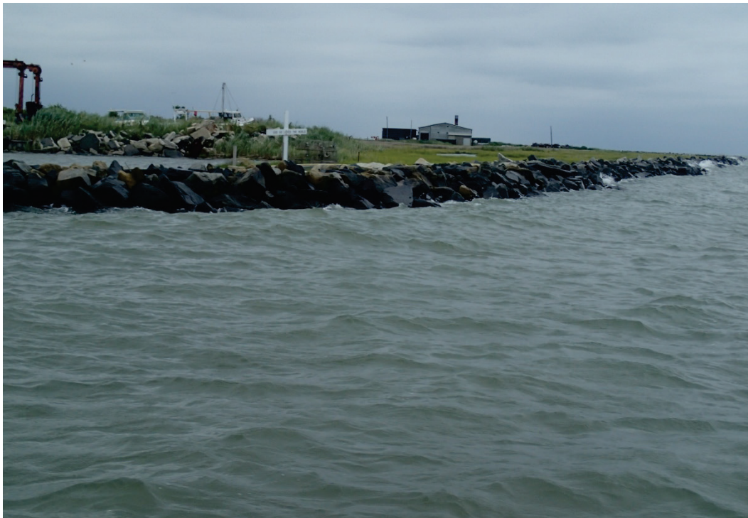
Figure 68. North end of revetment along the west side of Tangier Island.
